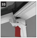
Fit the internal plastic cover by clipping in place.
