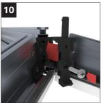
Secure in place using the ridgeLOCK fixing bracket over the left and right hand parts and bolt into the ridge. Repeat process at opposite end of the ridge.
