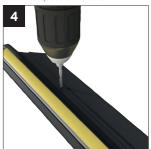
Drill 100mm from each end and drill a minimum of 4 holes at a Max of 400mm centres using appropriate clearance drill. Now take the eaves beam/rail and ensure correct number of bolts are slotted into eaves beam/rail
