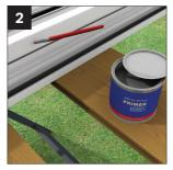
Ensure the surface is dry – apply a thin primer coat using a fine brush.
