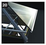
Lift glass units into place onto the eaves support trim and lower into place. Ensure that the glass contacts the gaskets on the glazing rafters and the ridge. Peel away protective film from glazing support.
